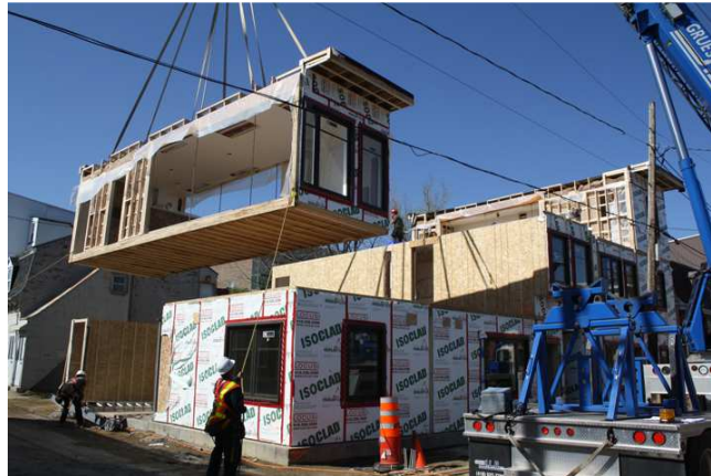
Photo 2: An example of modular construction
